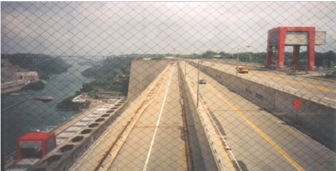
View north parkway lanes across Power Plant/Lewiston Road, top right
