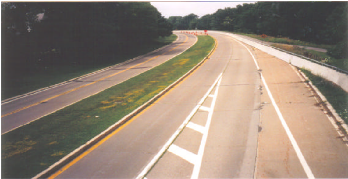
View south parkway lanes approaching Whirlpool State Park
